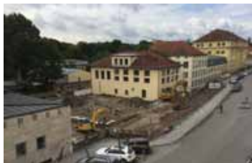
Construction site of the new Nano Institute
